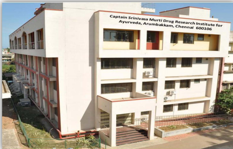
Premises of Captain Srinivasa Murti Research Institute for Ayurveda and Siddha Drug Development, Chennai
